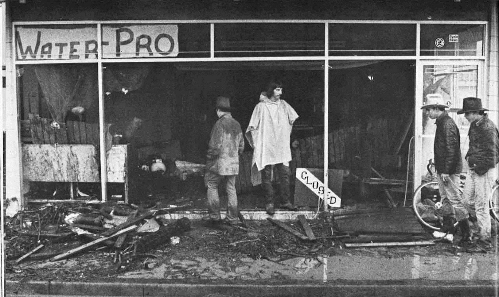
The Water-Pro on Pacific Street near Higuera was devastated.
